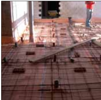
Installation of reinforced concrete.
