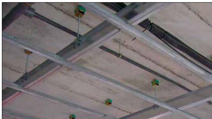
Application of an Akustik 4+Sylomer 30 type A.
