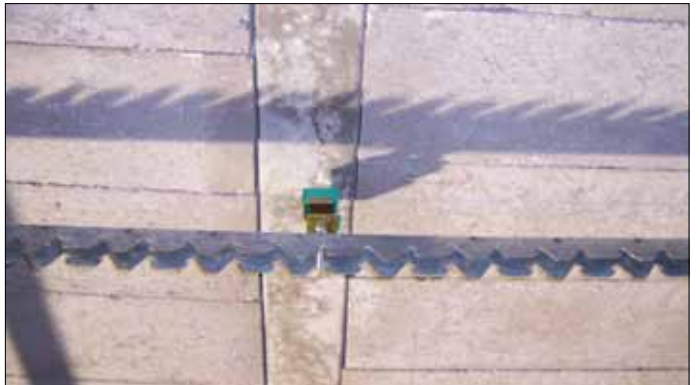
Application of Akustik+Sylomer mounts with different plasterboard beams.
