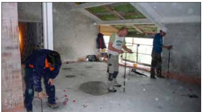
FZH mounts being levelled on a recording studio that is on the last floor of an Apartment block.
