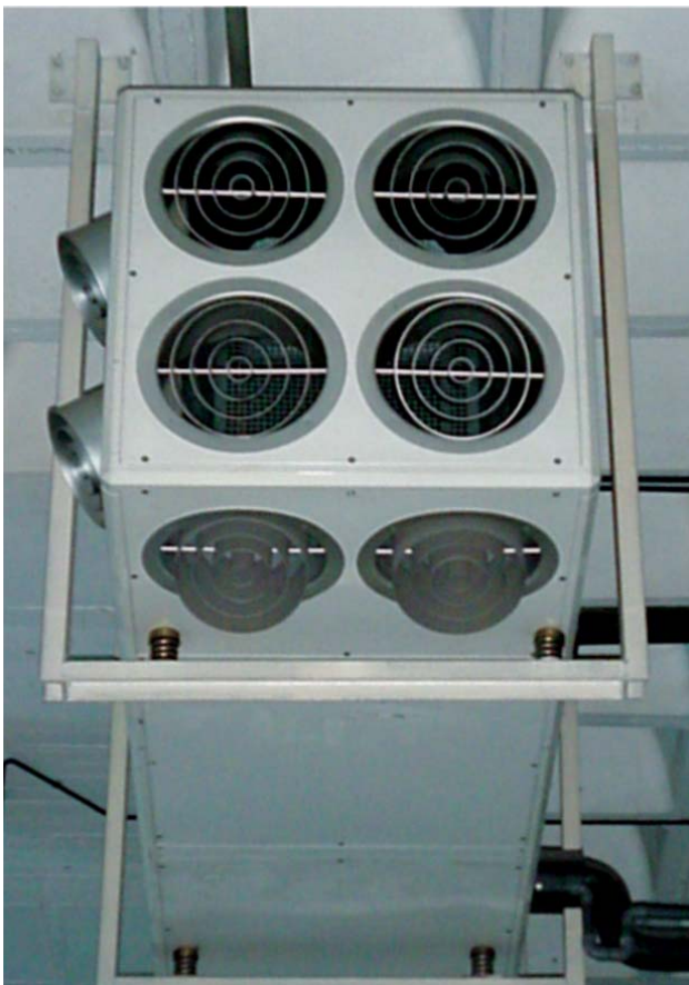
Ventilation system insulated with VIBRABSORBER®
